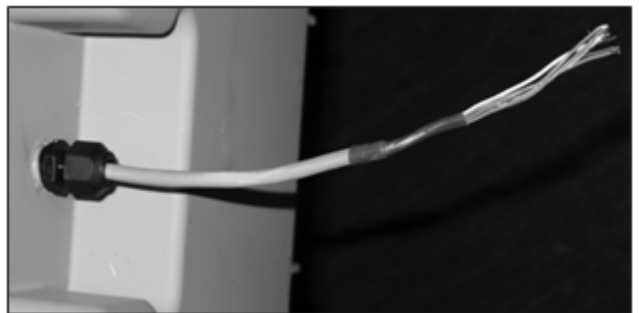
Figure 19: Loosen cable gland and extend the cable out of the gland
