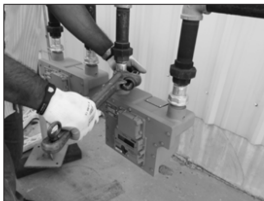
Figure 9: Use a pipe wrench to tighten swivel nuts
