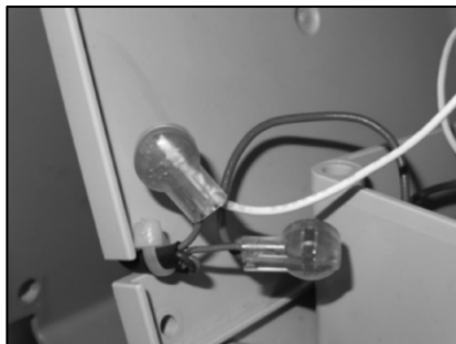
Figure 27: ERT cable properly routed through the back plate
