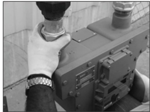
Figure 6: Connect meter ferrule into swivel nut on the gas supply side
