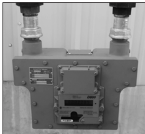
Figure 8: Meter placed in line
