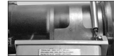
Figure 26 - Attach AMR to ETC bracket
