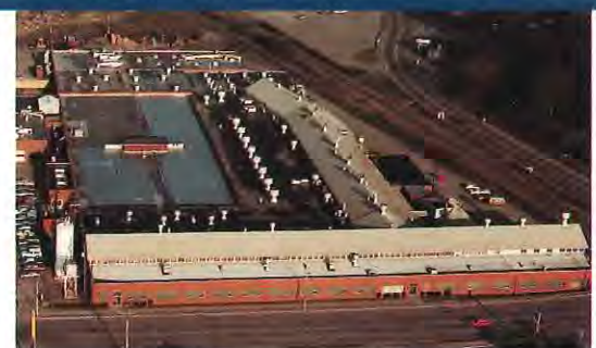
Sensus Metering Systems' headquarters in DuBois, Pennsylvania
